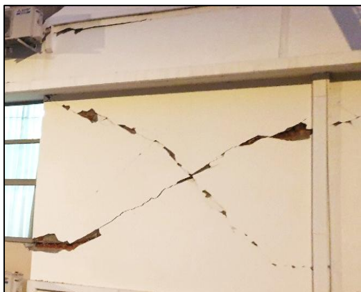
Figure 1.1 various types of cracks observed in masonry walls
