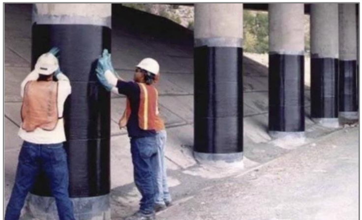
Figure 3.5 CFRP Strengthening
