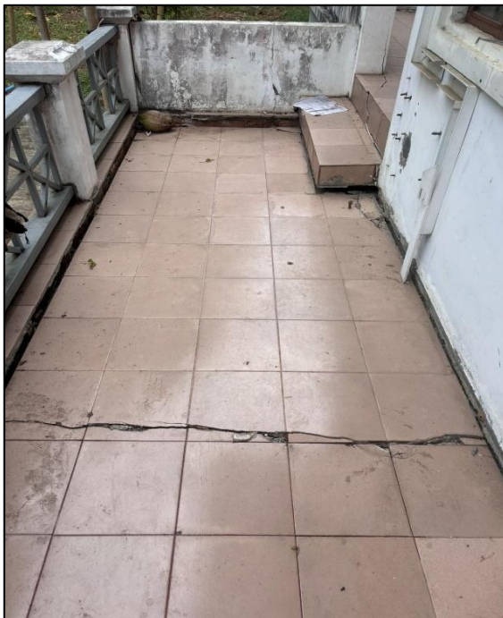
Figure 1.10 Settlement of Ground floor
