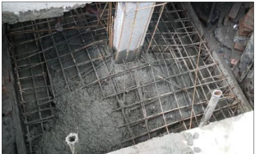
Figure 2.9 Strengthening of Footing
