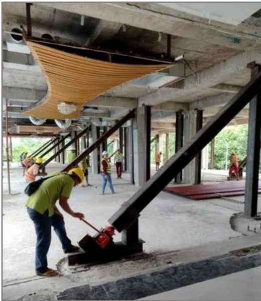
Figure 3.3 Temporary Bracing inclined strut and Strengthening with Bracing
