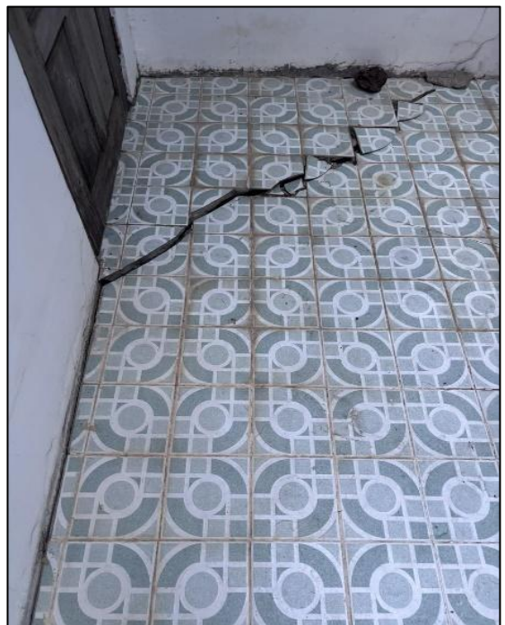
Figure 1.10 Settlement of Ground floor
